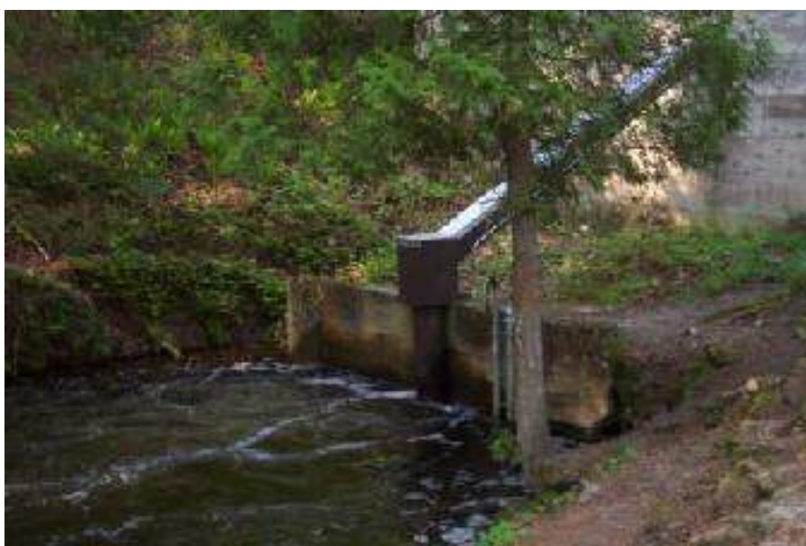
Photo 10. Closeup view of minimum flow monitoring. Minimum flow is 50 cfs from the powerhouse.
