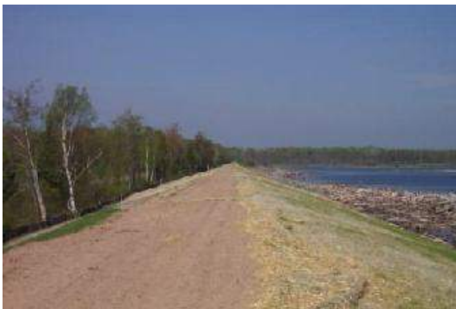
Photo 17. The South Levee, which is an earthen dike, creates the divide between the Lake Superior (on the right side of the photo) and Lake Michigan (on the left side of the photo) drainage basins.
