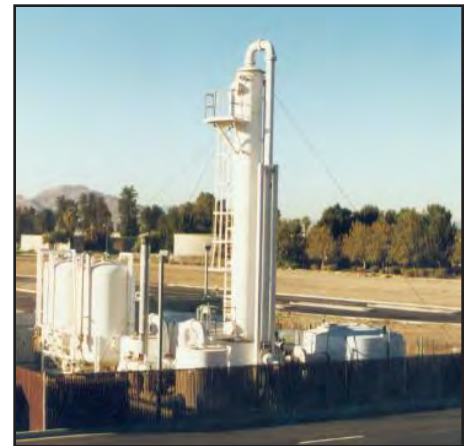
This pump and treat system was used at the former Norton AFB, Calif.
