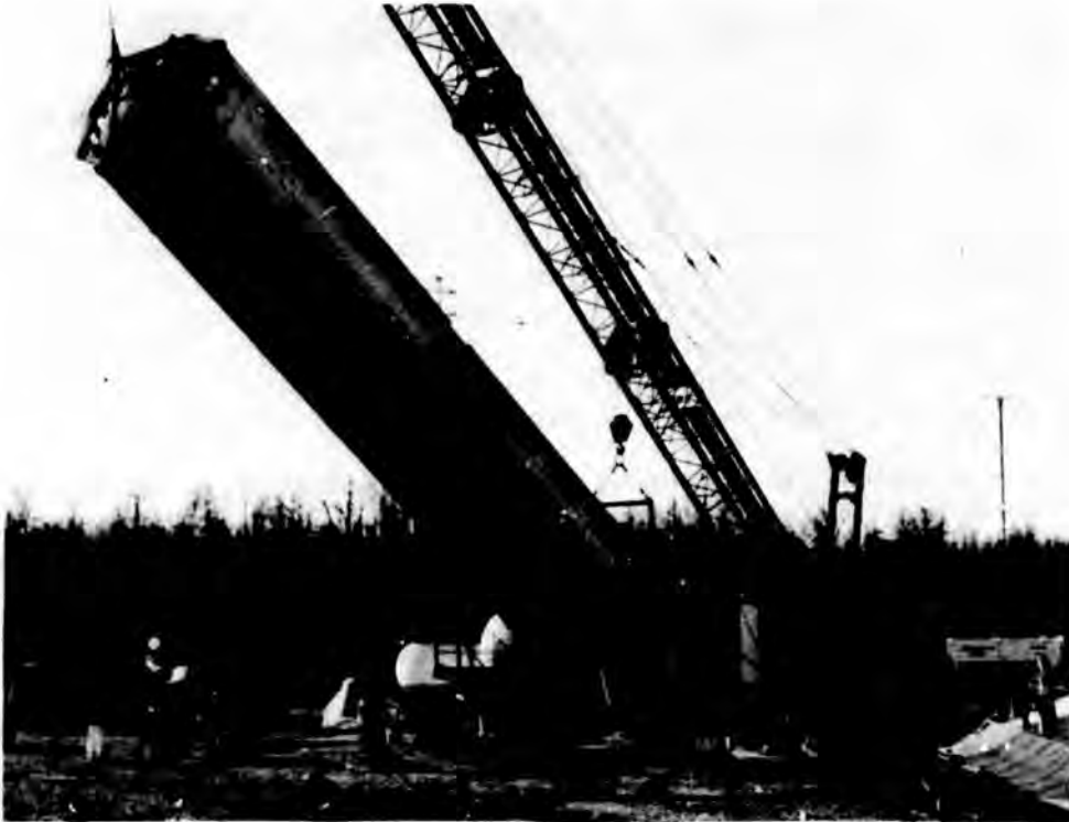
Titan II after removal from silo
