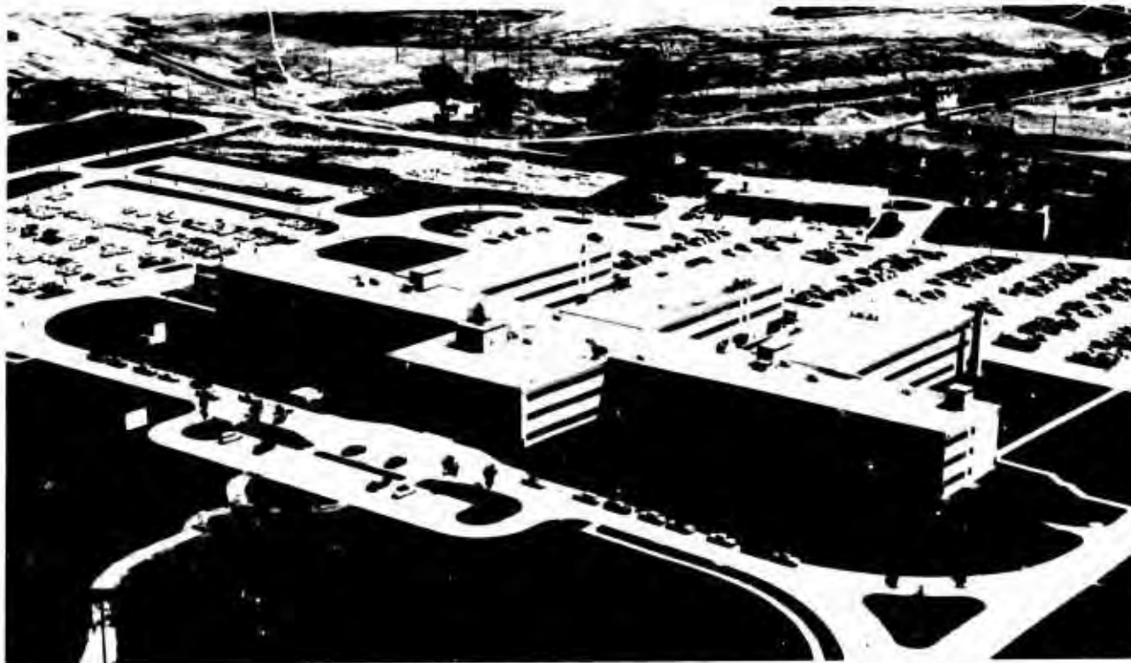
New Headquarters SAC Building, Offutt AFB, Nebraska, 1957
