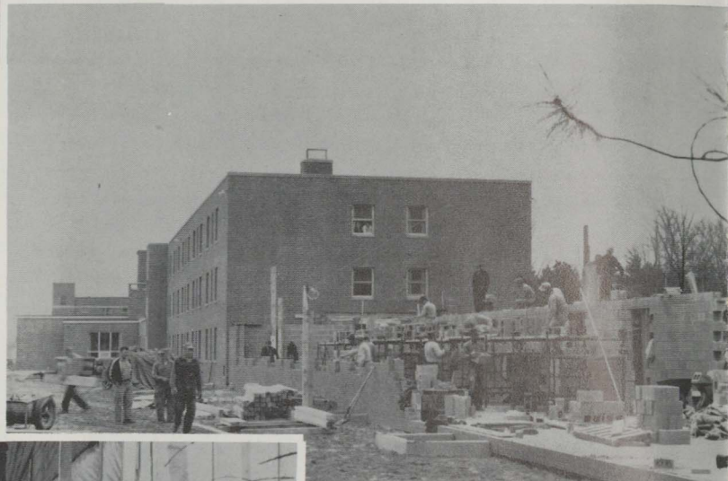
And a new addition growing on Spooner Hall, to be open next fall.
