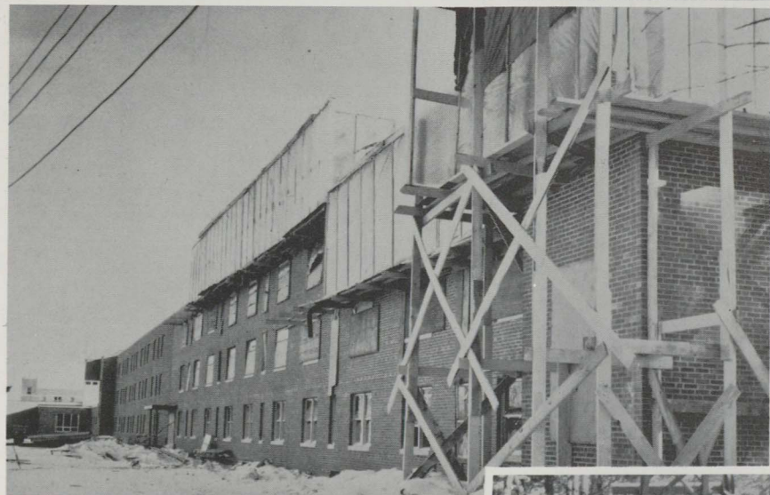
Construction in progress
