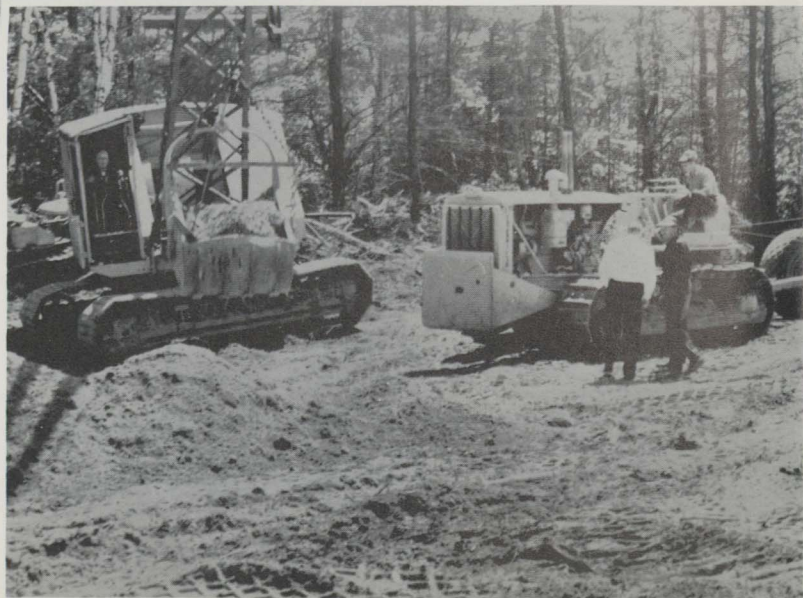
And more land being cleared for more buildings
