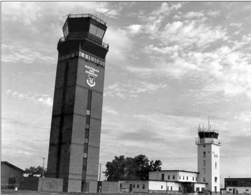
In 1992 at Whiteman Air Force Base, Missouri, the newly constructed aircraft control tower dwarfed the old one and symbolized the return of a flying mission to the base.
